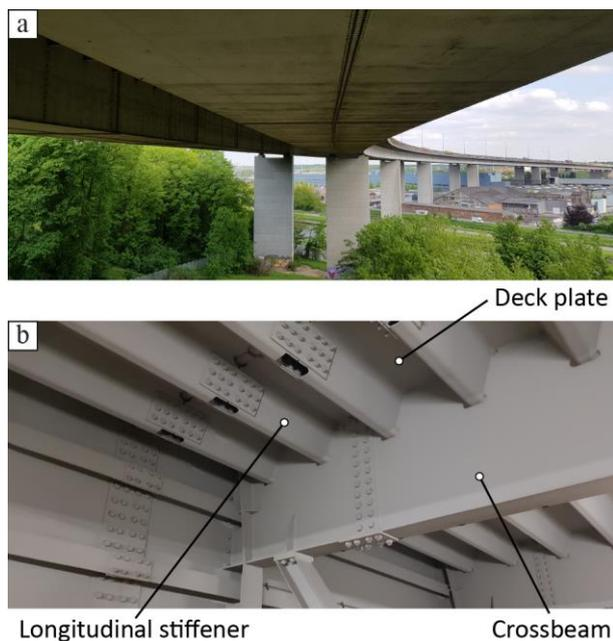
Figure 1. Viaduct of Vilvoorde. (a) Closed box girder seen from below; (b) OSD details inside the box girder
